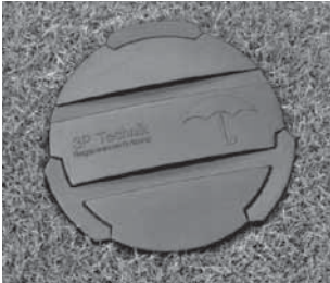
1. View of the lid of the filter which has to be opened at first.
